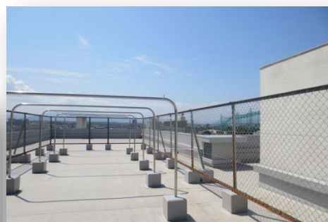
↑Roof (for laundry)
